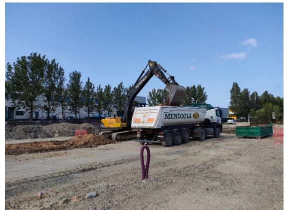
Figure 19. Loading of lorries for the reuse of soil at authorised landfill sites.
