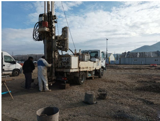
Figure 15. Drilling of piezometric boreholes
