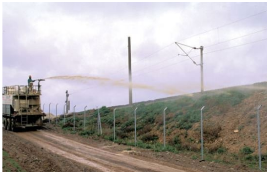
Figure 25. Fire protection measures on tracksides.
