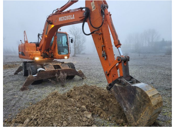
Figure 18. Execution of test pits for sample collection.
