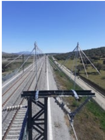
Figure 26. Anti-nesting devices on the overhead wires Madrid-Extremadura Line
