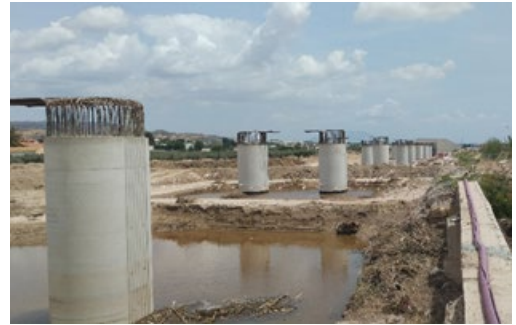
Figure 10. Rainwater is collected in the pile cap of the Totana-Lorca viaduct.
