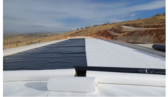
Figure 39. Platform Waterproofing Before Sub-ballast Installation
