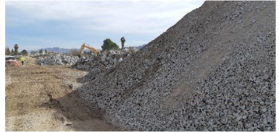
Figure 18. Recycled aggregates prepared for use on site
