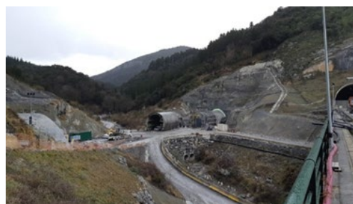
Figure 19. General view of East and West Udalaiz's tunnels during the construction phase (MEB worksite, Sector 2)
