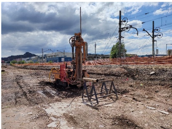
Figure 25. General view of the smelter site during drilling of the boreholes
