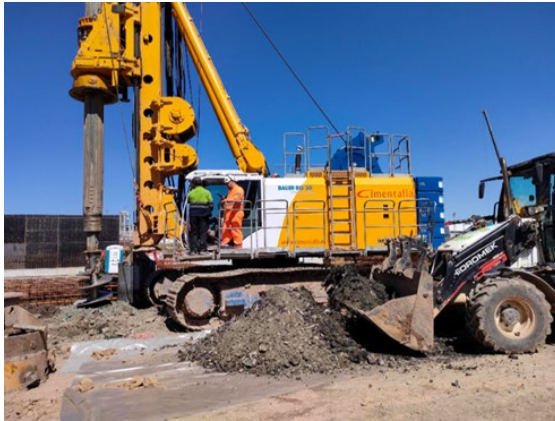
Figure 22. Collection of waste from pile drilling at the foot of the machine
