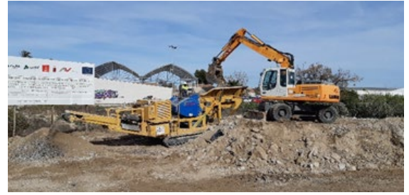
Figure 17. Crushing plant located on the Nonduermas Underground works
