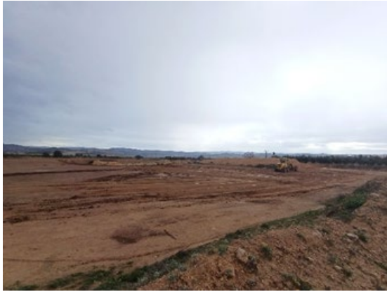
Figure 13. Mining pit levelled and conditioned to the level of the adjacent plots
