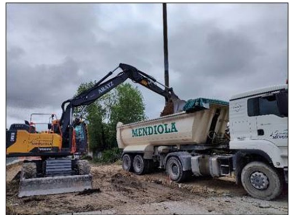
Figure 28. Loading of lorries for the reuse of soil at authorised landfill sites
