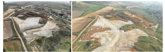
Figure 16. Current state of the quarry once filling with soil from the construction site has begun
