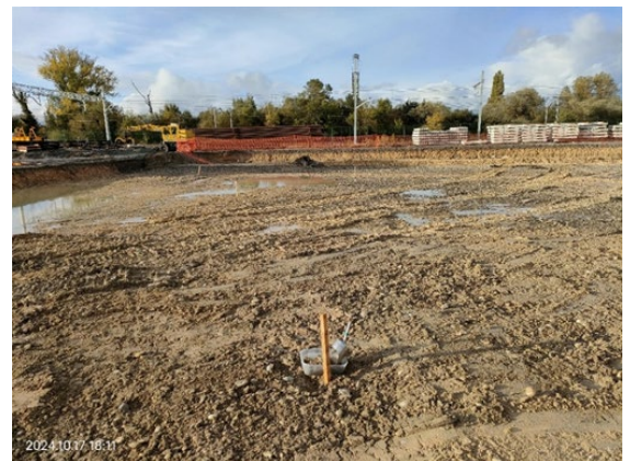
Figure 29. Sampling of remaining soil
