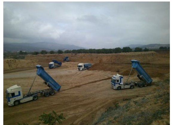
Figure 12. Backfilling work during the restoration of the mining void
