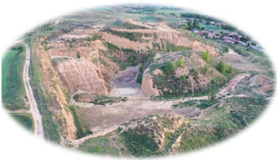
Figure 14. Condition of the quarry before work commenced
