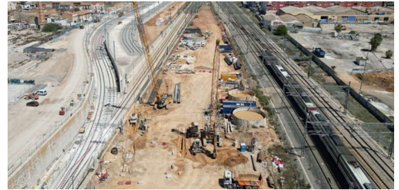
Figure 11. Aerial view of the bentonite slurry deposits used during the construction of the slurry walls
