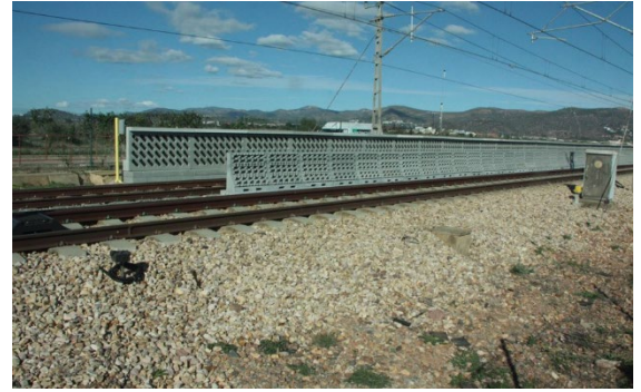
Figure 36. Testing of mini and micro acoustic barriers on the railway network
