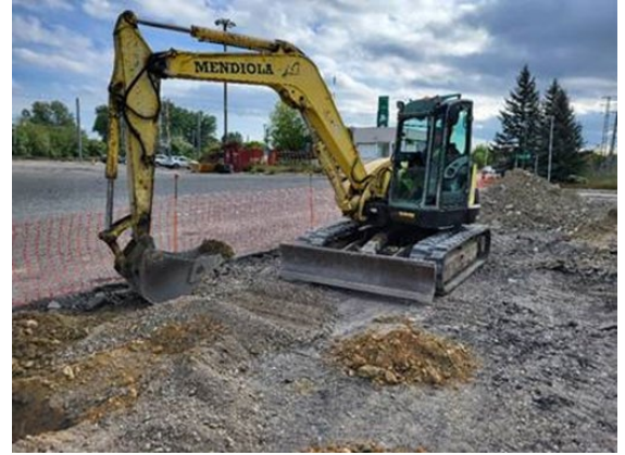
Figure 27. Execution of test pits for sample collection
