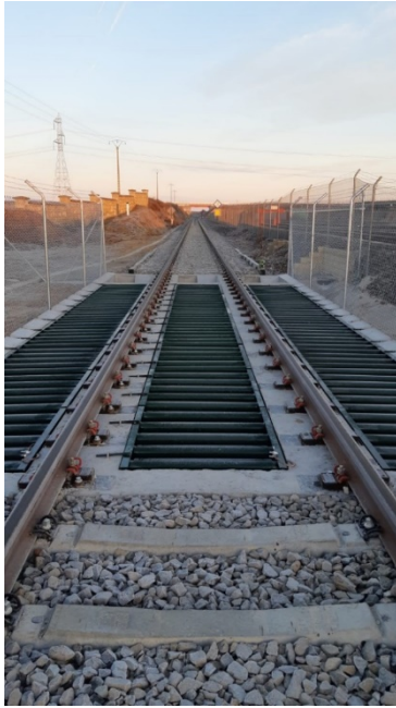
Figure 40. View of the completed Canadian crossing
