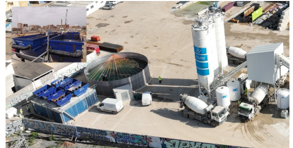
Figure 9. Aerial view of the water deposits and decanters installed next to the concrete plant
