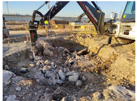
Figure 24. Dismantling of Logistics Operator 1
