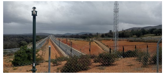
Figure 44. Infrared camera used in the video surveillance system
