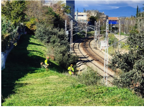
Figure 37. Fire protection measures on tracksides
